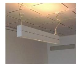
Figure 3. Luminaire with direct and indirect light output.
